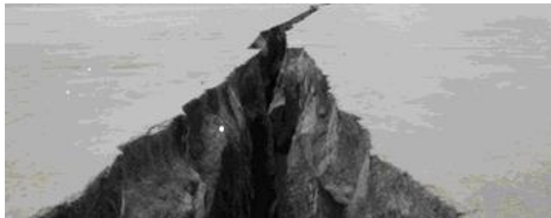
Fig. 9 – Tate Modern Gallery in London enter the galleries giant turbine hall, confronted are the disturbing sight of a giant crack. Starting as a small fissure, the 167 m fracture grows wider and deeper as it snakes the entire length of the hall.
